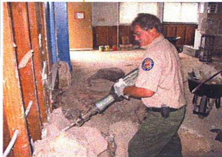
Bob Scholfield demolishing old tide pool exhibit
